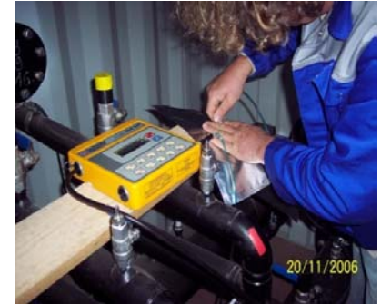
III. 3 Measurement in the gas collection station [DAS-IB GmbH, 2009]
