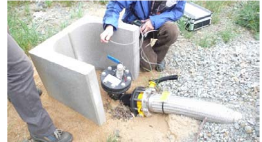
III.2 Measurement at the wellhead [DAS-IB GmbH, 2009]
